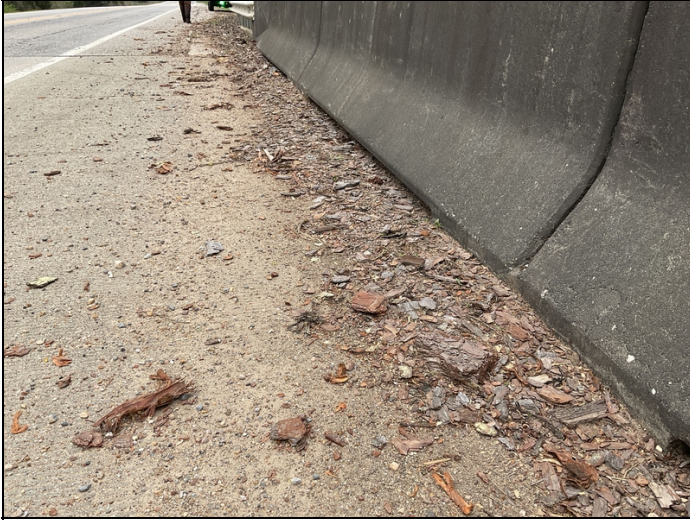
Deck washing needed, Both right and left sides of bridge deck have debris blocking drains, Typical in all spans
