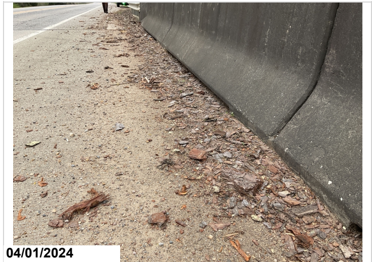
Deck washing needed, Both right and left sides of bridge deck have debris blocking drains, Typical in all spans
