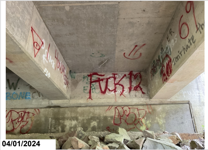
Span 1, Bay 1, Efflorescence to undersurface of deck, CS2
