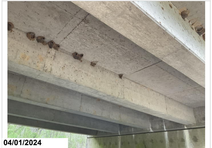
Concrete t-beams, Typical of all spans
