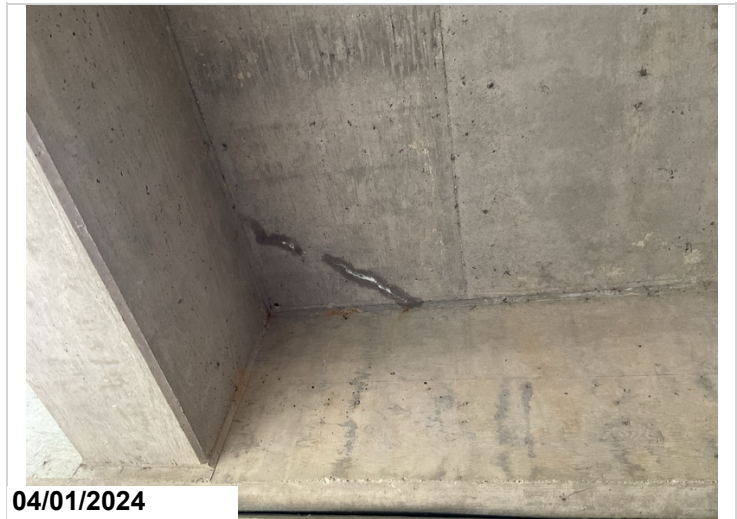
Span 4, Bay 4, Efflorescence to undersurface of deck, CS2
