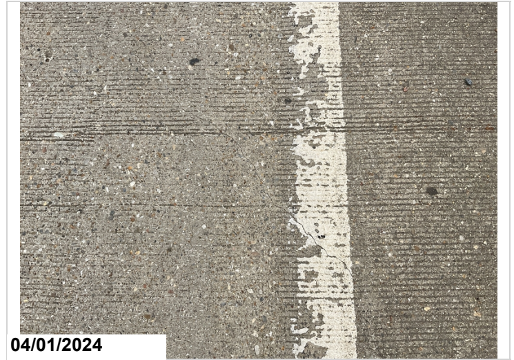
Span 4, Rt side, Deck cracking, Typical of all spans, CS2
