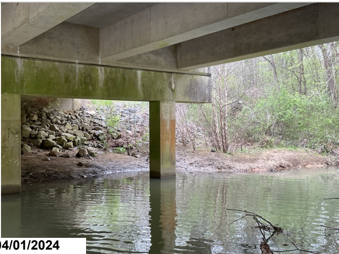
Bent 2, Looking back, Efflorescence to left side of cap above column 1. CS2
