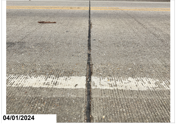
Bent 4, Loss of seal adhesion, Typical of bents 2, 3, and 4. CS3
