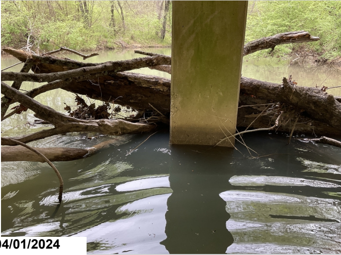
Bent 3, Column 1 spill, CS2.
