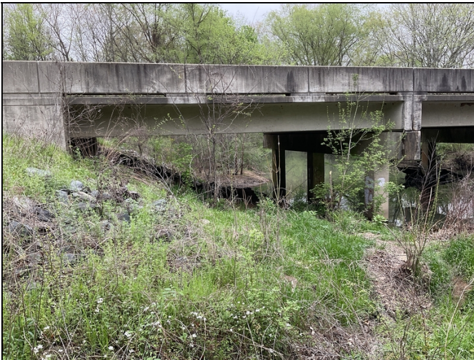
Span 1, Right side, Trees and vegetation need removed
