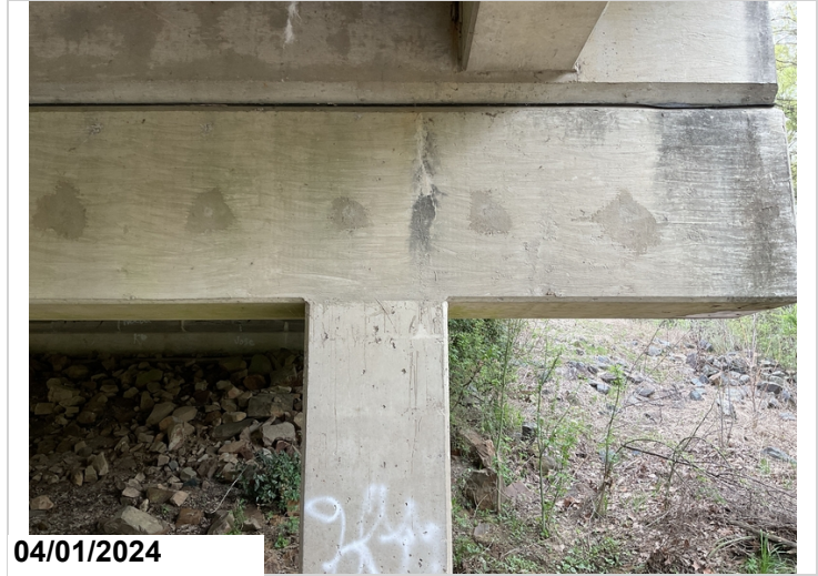
Bent 4, Looking ahead, Efflorescence to right side of cap above column 3. CS2
