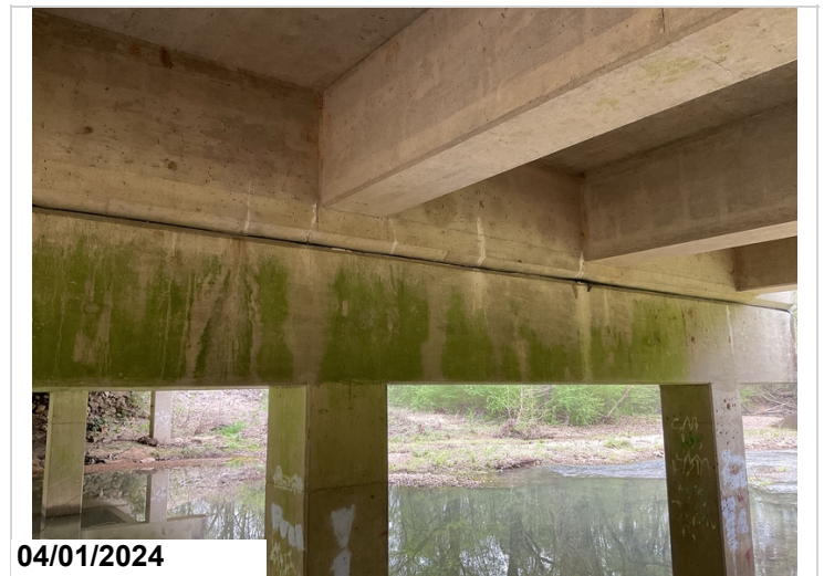
Majority of efflorescence is on concrete diaphragm between beams at bents Efflorescence is found on the concrete diaphragms between beams at all bents.
