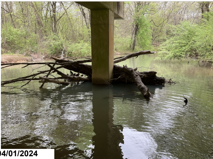
Logs and debris against bent 3 column 1.
