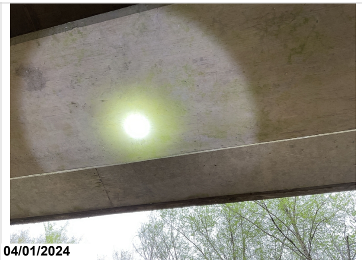
Span 1, Beam 1, Minor hairline cracking that is unsealed, CS2
