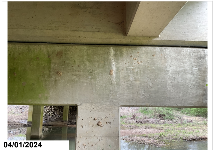
Bent 2, Looking ahead, Efflorescence to right side of cap above column 3. CS2
