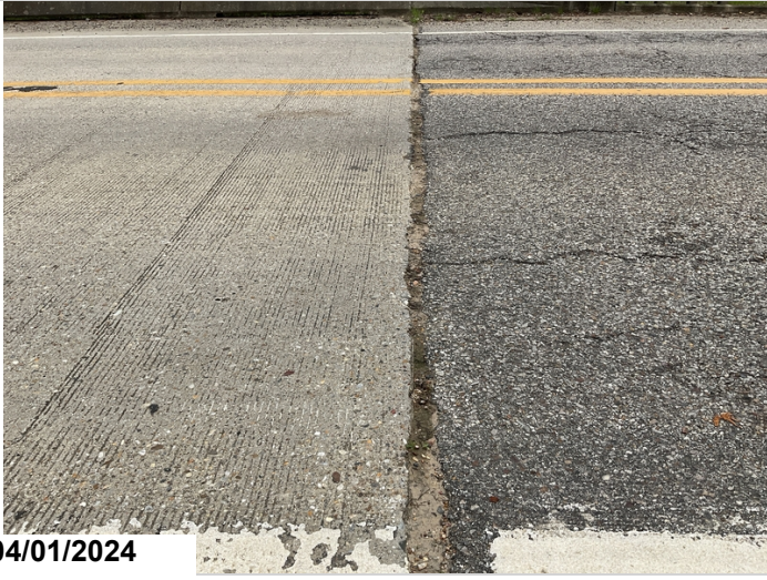
Bent 5, Debris impactation, Typical of bents 1 and 5. CS3
